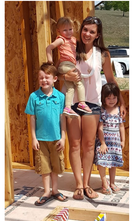
Janelle Poulsen pauses during the wall raising with her children Rowen, Benna and Qwynn.
