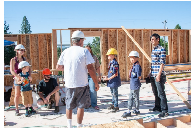
Construction Supervisor Dave Stradley paused construction to give a tour to Pack 323 (Moscow) Arrow of Light Den members.
