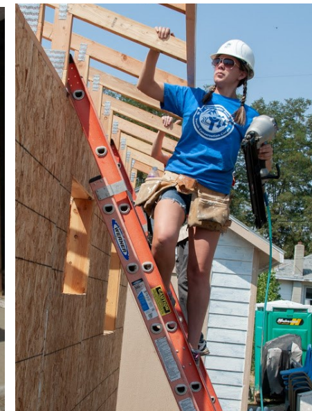
Janelle Poulsen installing subfascia.
