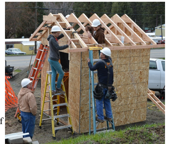
Scouts installing the roof trusses supervised by Dave Stradley and Dave Ostrom.
