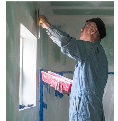
Codger Crew Member Bert Smith mudding drywall
