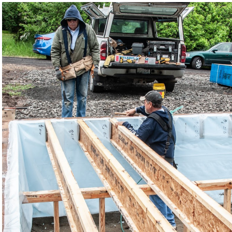
Codger Crew member Marc Ratzlaff helping Dave Stradley install I-joists to support the floor.
