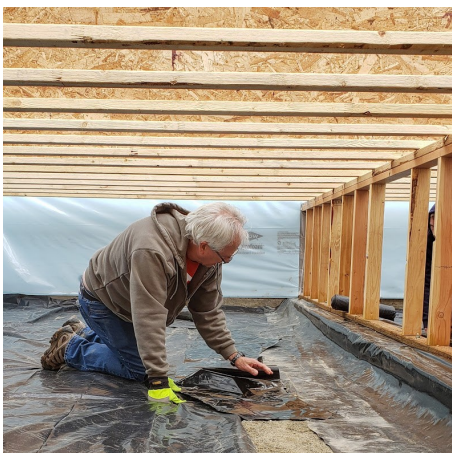
Volunteer Jason Franklin installing vapor barrier under the I-joists.
