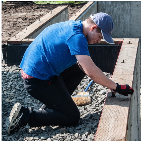
Volunteer Corey Franklin installing mudsill.
