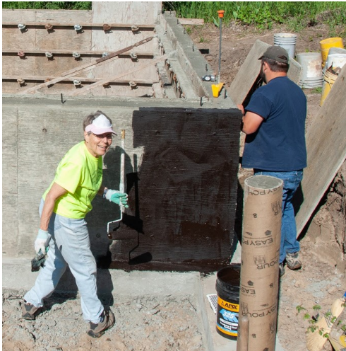
Codger Crew Member Carolyn Adam and Volunteer Alex Gisler apply waterproofing to the exterior of the foundation wall.
