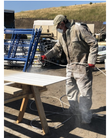
Construction Supervisor Dave Stradley spray painting siding
