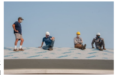
Dave Stradley and Codgers wait for shingles to be delivered.
