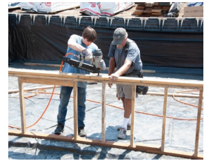
Construction Supervisor Dave Stradley helps a Fairfield Inn volunteer secure the top plate to the crawl space wall.
