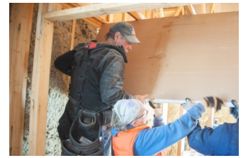
Dave Stradley installs sheetrock at the Hansen home with Chris Montfort.
