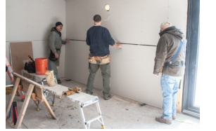
Bert Smith, Tim Halvorson and Marc Ratzlaff place drywall in the Hansen kitchen.
