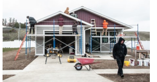
Volunteers touch up exterior paint.
