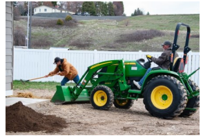
Dave Stradley and Jacob Maurin preparing the yard for hydroseeding.
