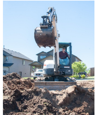
Rex Brown running the excavator.
