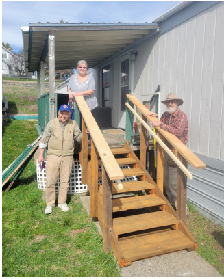
Stair installation in Colfax
