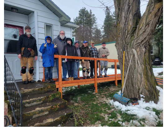
Ramp installation in Palouse
