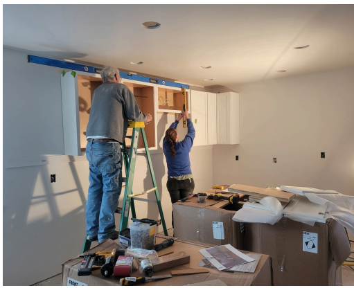
Cabinet installation in Palouse
