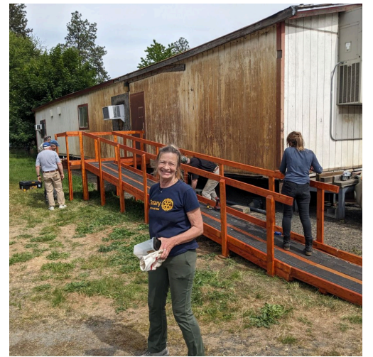
Recent ramp installation in Orofino
