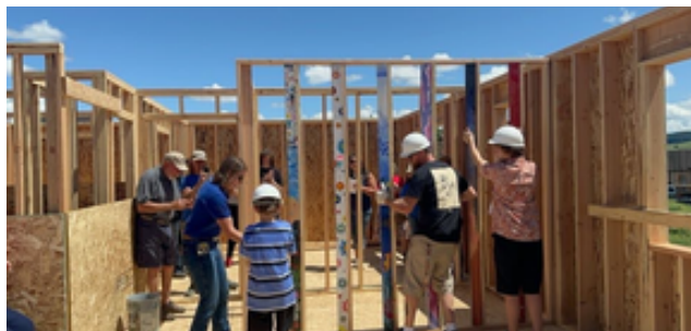
Jake and his family raising one of the final walls in their future home last June
