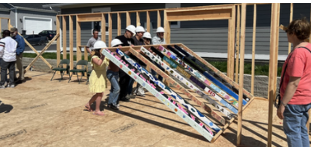
Kaylee and her family raising one of the final walls in their future home last April
